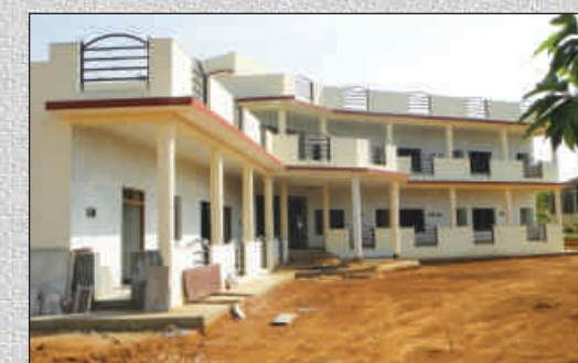
New laboratory building coming up at Attur
